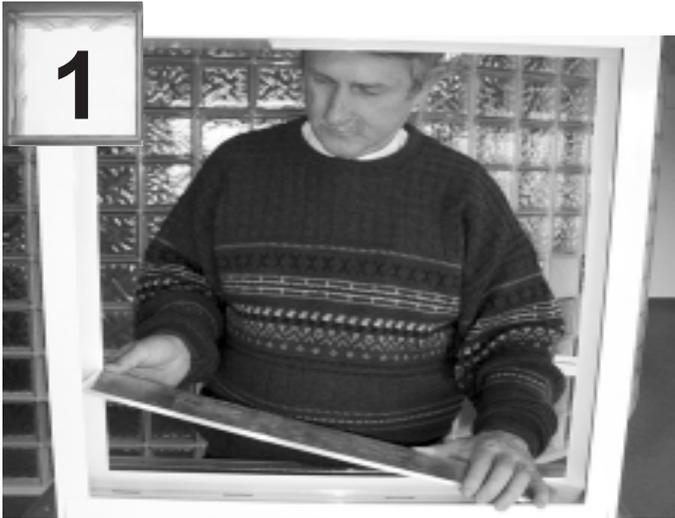
Place sill infill in bottom of frame.
